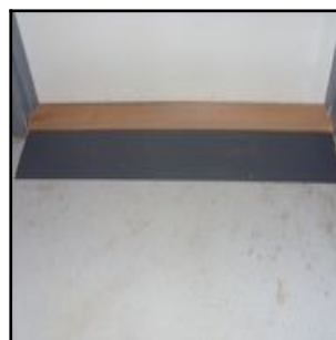
Ramp on site
